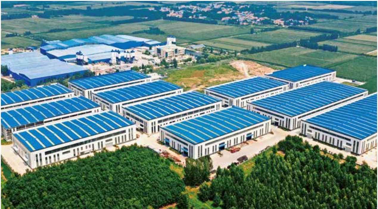
Shandong Fuding Industrial Park
